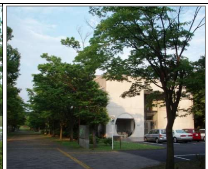
Building No. 13 (Physical Education Research Building)
