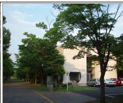
Building No. 13 (Physical Education Research Building)
