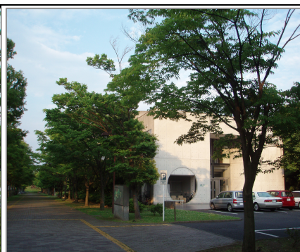
Building No. 13 (Physical Education Research Building)
