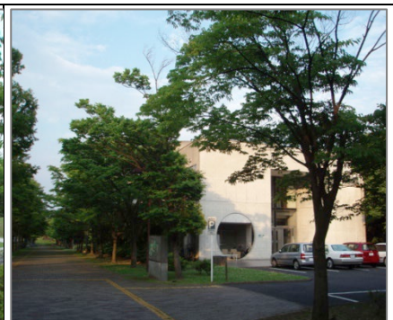
Building No. 13 (Physical Education Research Building)
