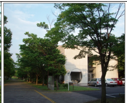
Building No. 13 (Physical Education Research Building)
