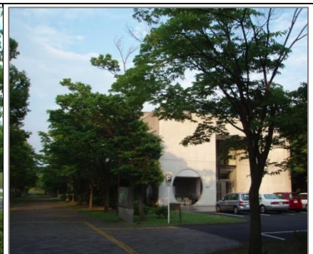
Building No. 13 (Physical Education Research Building)
